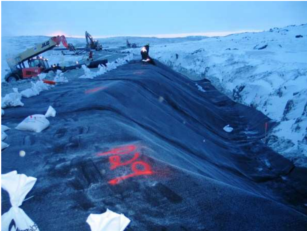
Photo 9: HDPE liner placement
