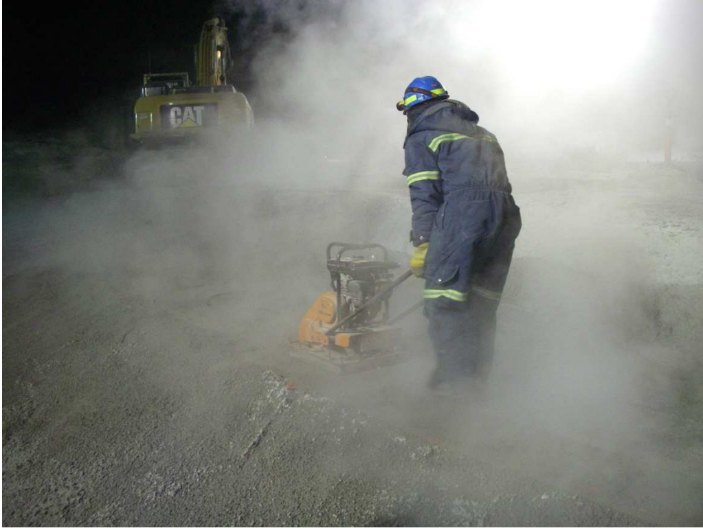
Photo 13: Small compactor being used on the core material.
