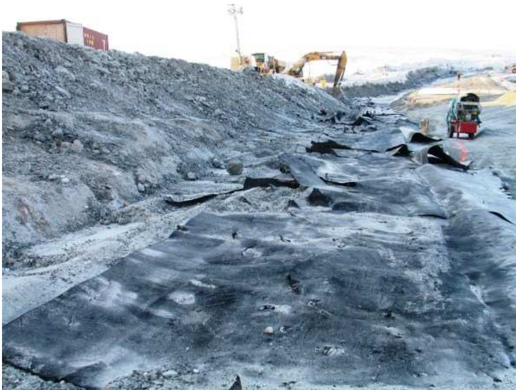
Photos 4: ROQ removed from top of HDPE facing south (morning view)
