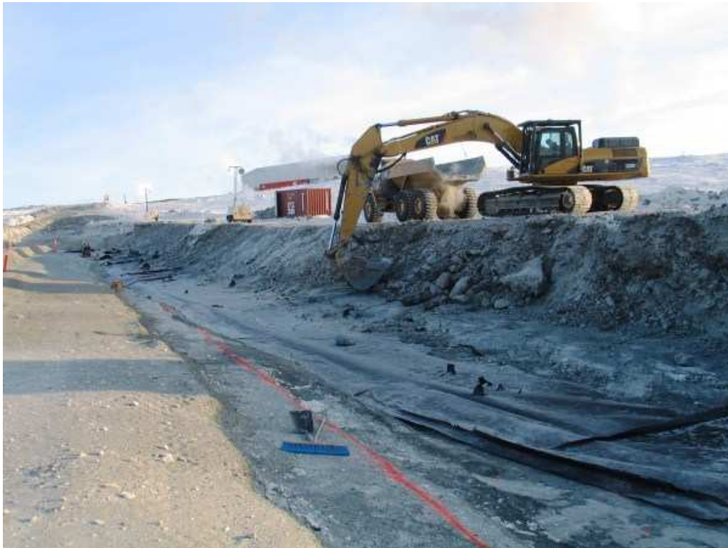
Photo 3: Excavator reshaping ROQ slopes and cleaning above GCL at north end.
