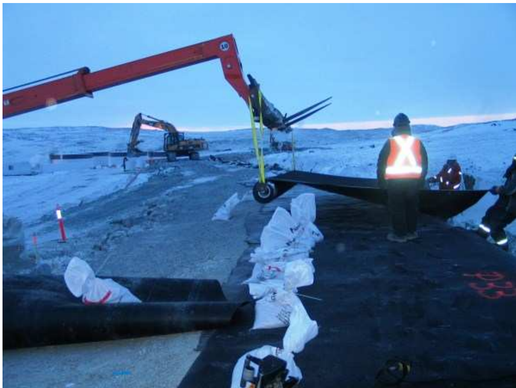
Photo 10: Layfield placing HDPE
