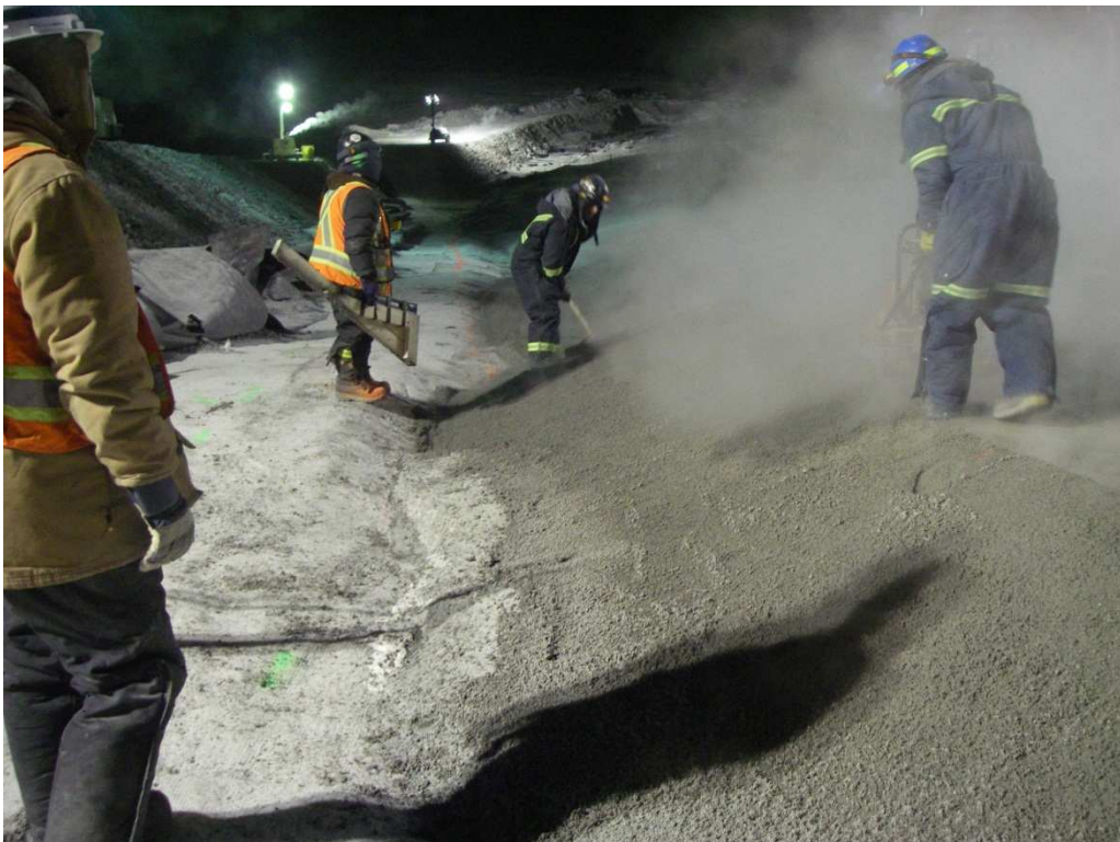
Photo 14: The 2.5H:1V slope being finished using rakes and shovels.
