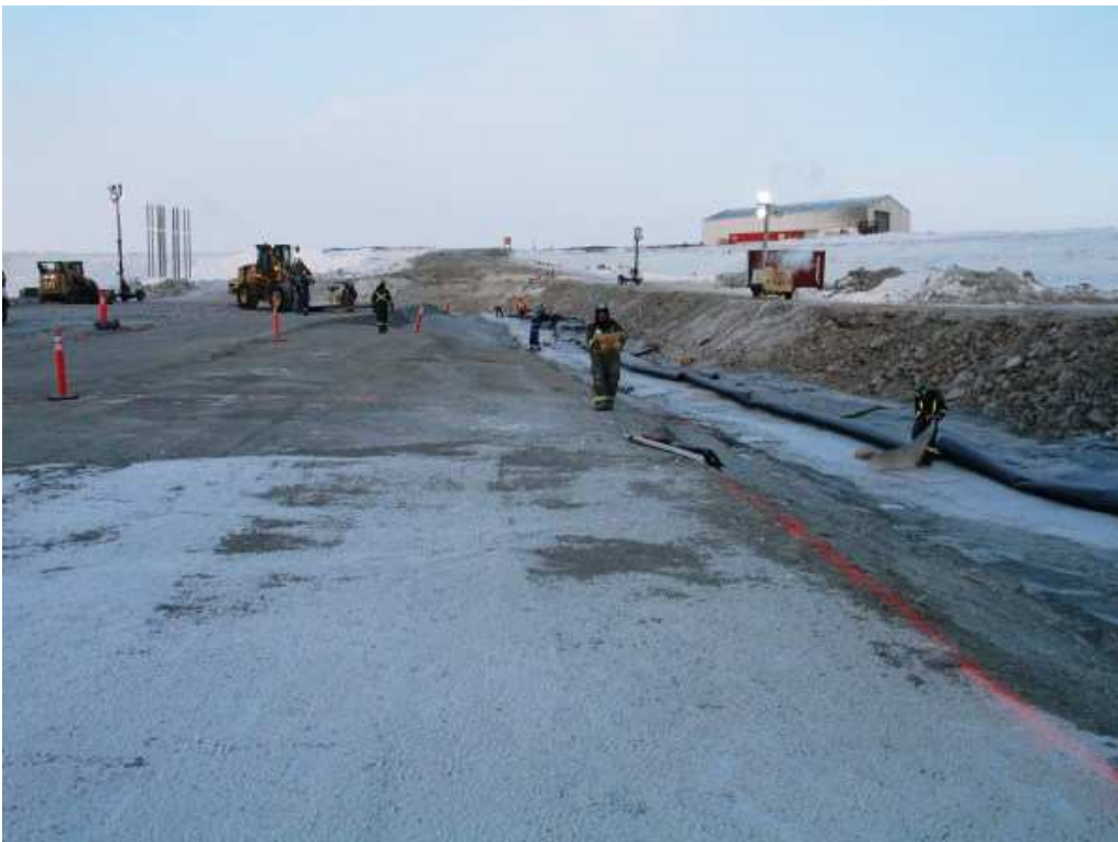
Photo 6: labourers patching GCL north end.
