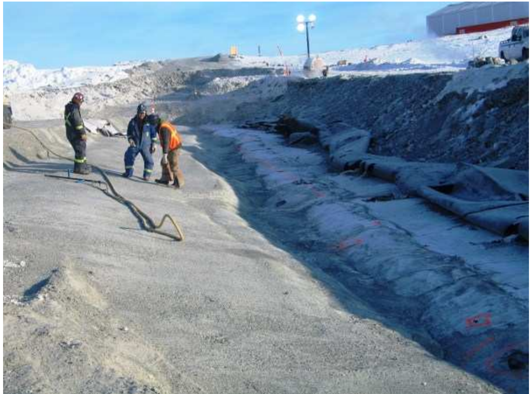
Photo 2: North east corner after cleaning with air compressor.
